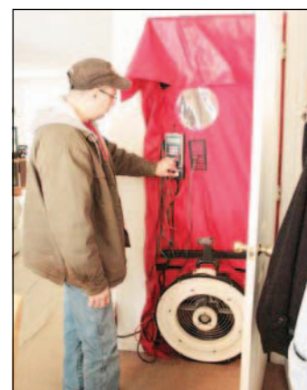
Paul Chalifour, an energy auditor with Southern New Hampshire Services, demonstrates how a blower door works.
